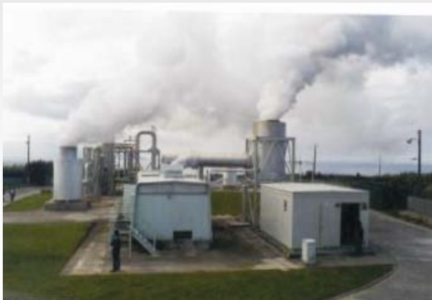
Pico Vermelho, Azores (direct-intake, dry steam)
