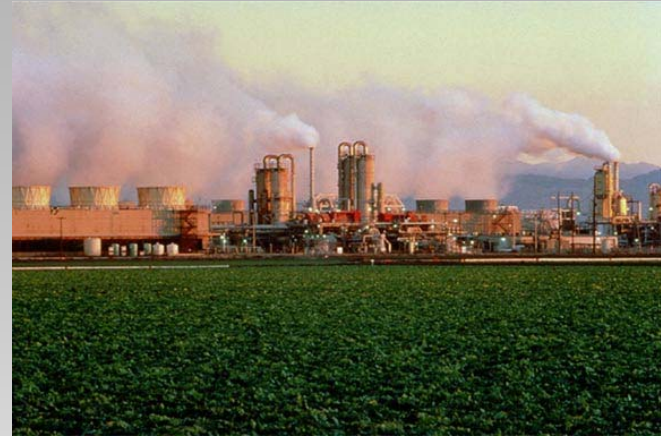
Imperial Valley, USA (wet steam, double flash)
