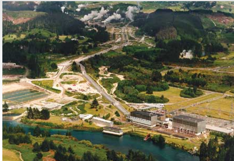
Wairakei, New Zealand (wet steam, triple flash)
